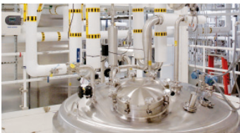
Biologics Manufacturing Facility, Maryland
