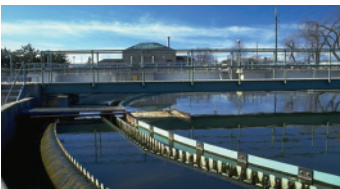
Traverse City Regional Wastewater Treatment Plant, Michigan
