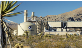
Silverhawk Power Station, Nevada
