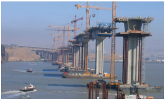
Benicia-Martinez Bridge, California
