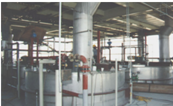
Rhodia New Fine Chemicals Plant, Mexico
