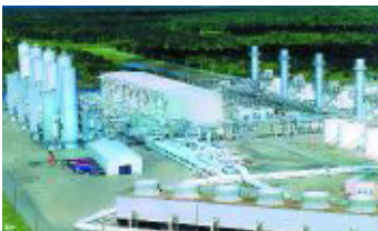
PEMEX Refinery Upgrade, Mexico
