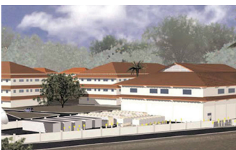
Telecarrier Data Center, Panama
