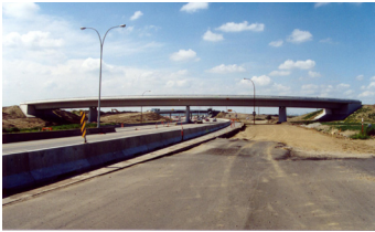
Barlow Trail/Deerfoot Trail Interchange, Alberta
