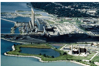
Lakeview Water Treatment Plant, Ontario
