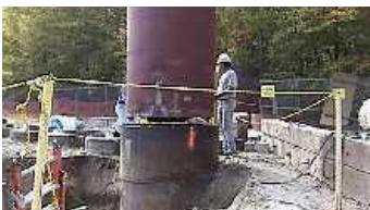
Bruce Nuclear Power Facility, Ontario
