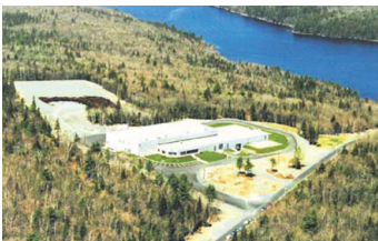
Lake Major Water Treatment Plant, Nova Scotia
