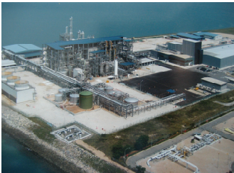
Turnkey EPCM Services for Chemical Process Plant on Jurong Island
