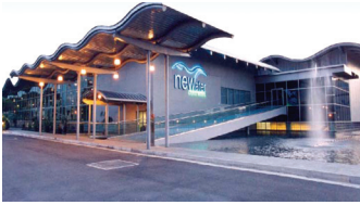
PUB Bedok, Kranji, Seletar, and Changi NEWater Plants and Visitor Centre
