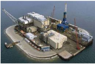
Engineering, Construction, and Startup British Petroleum, Alaska
