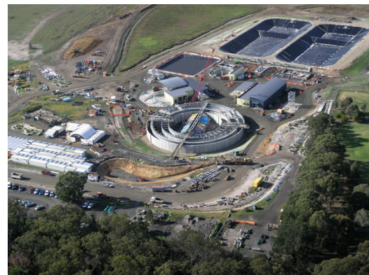
Maryvale Treatment Plant under construction (2008)
